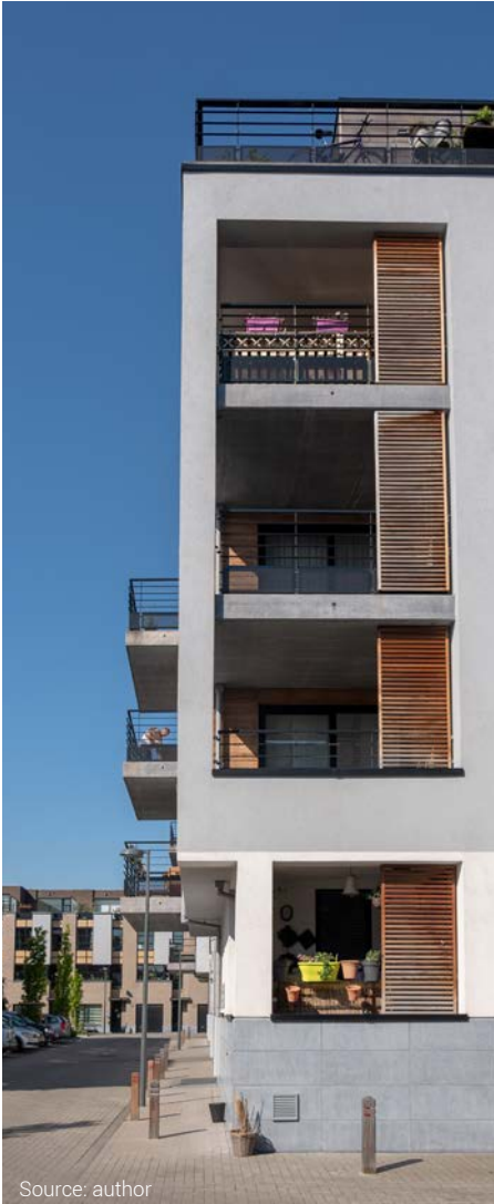
Figure 17 | Throughout the project, terraces are of the loggia-type. As opposed to conventional protruding terraces, the loggias are situated within the buildings main structure and are thus less exposed to public space.
