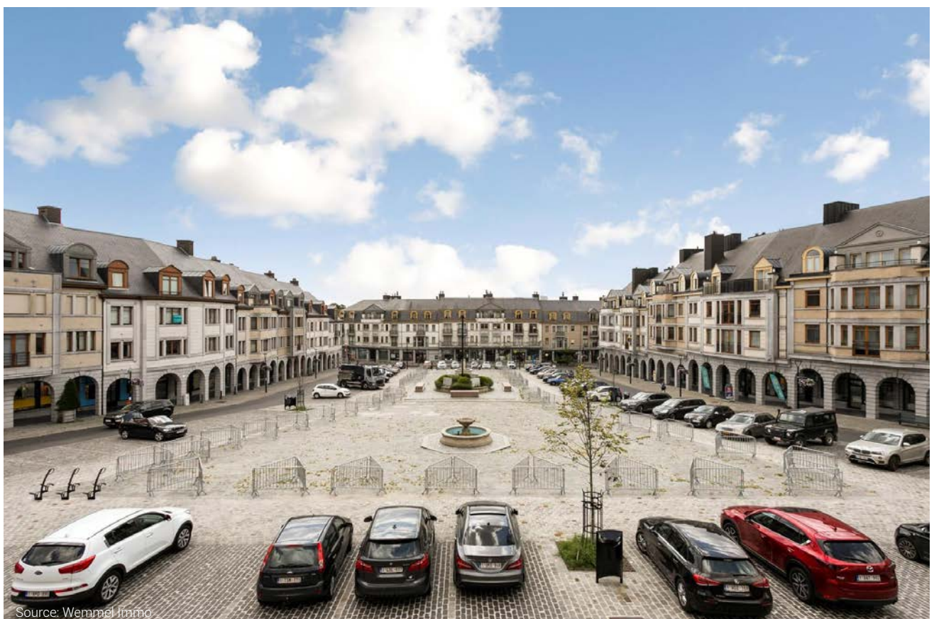
Figure 44 | The middle of the square, fenced off for renovation, will provide additional car spaces.
